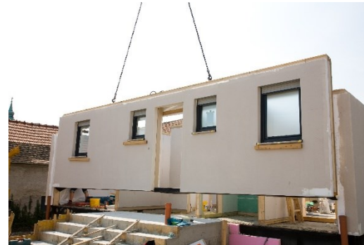
Transforming construction (up to £170m)
